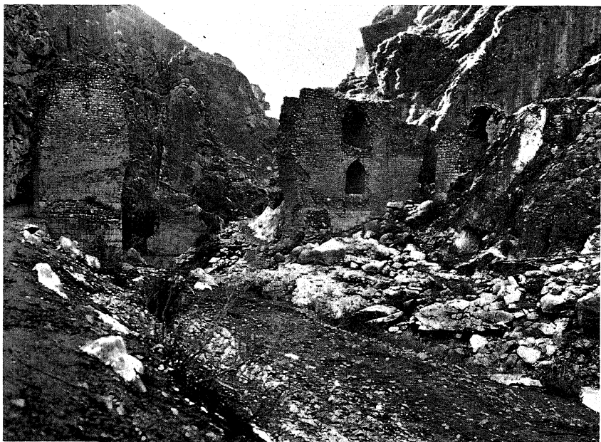
83. RUINED BRIDGE ACROSS KĀSHGĀN RIVER AT KALHŪR, PĪSH-I-KŌH
